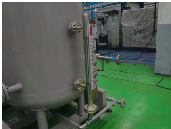
Magnetic plate level meter: the scene display is clear, far-transmission level alarm
