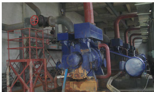
Shanxi Dongling Lead and Zinc Smelting Co., Ltd.
